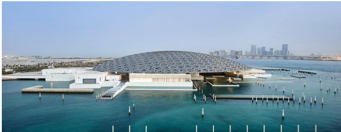
Figure 1: Ariel view of Louvre Abu Dhabi
