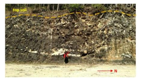
Figure 5. The parking lot in Pindul Cave provided for the tourists is located aside from a steep slope with no engineering that can support the slope stability.
